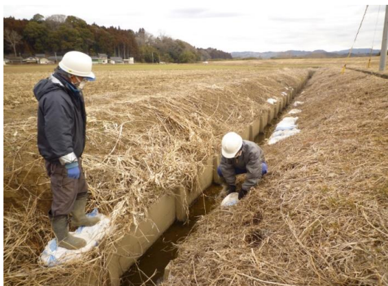
・水路の軽微な補修 (裏込め材の充填)
